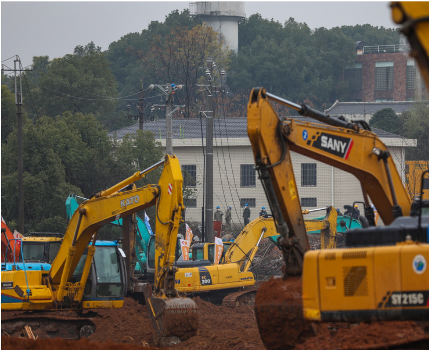
epa08157639 People work at the construction site of a field hospital in Wuhan, Hubei province, China, 24 January 2020. The hospital is expected to be completed by 03 February 2020 to cope with the increasing number of people affected by the coronavirus. The coronavirus has so far claimed 25 lives and infected more than 800 others, according to media reports. The virus has spread to Thailand, South Korea, Japan, Singapore and Taiwan. EPA/YUAN ZHENG CHINA OUT
